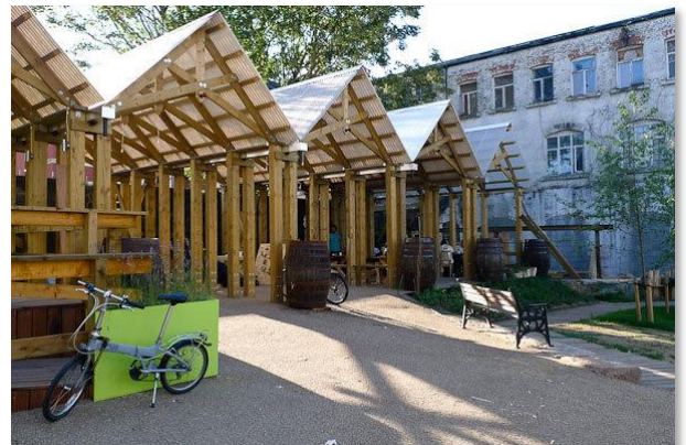
Figure 15: Simple timber oversail structure for modular units
